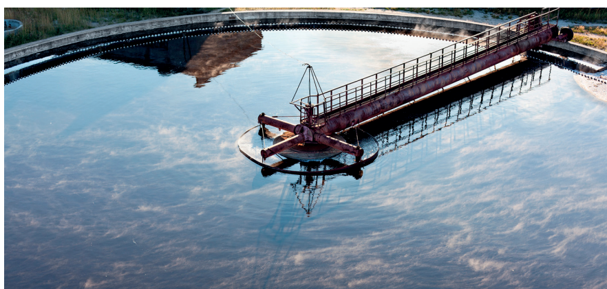
Plant optimisation is at the heart of wastewater treatment resilience
