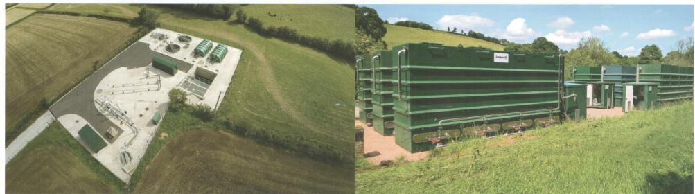
This separation appears logical as both solutions essentially perform the same task, removing BOD and ammonia from wastewaters for small populations of up to 3000 PE However there are persuasive reasons why it is worth considering a mix of both, tailoring solutions for the situations to which they are best suited.
