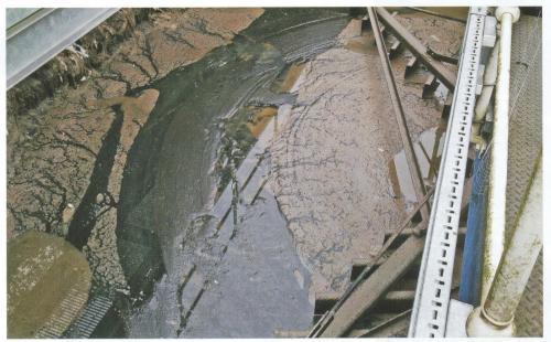
investigation, the Company found that the plant had not been running efficiently for years, leading to a massive grit build-up downstream that had compromised biofilters, many pumps and other critical plant. Following refurbishment and commissioning, including plant optimisation, the works is now running far more efficiently.
