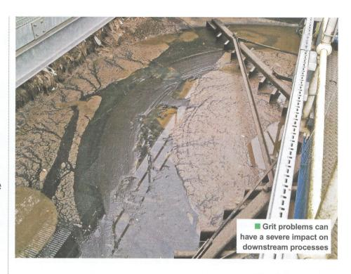
Grit in downstream treatment systems also reduces the available treatment volume and process efficiency. This affects final effluent quality, the amount of energy required to achieve the works' discharge requirements, and the efficient operation of sludge digestion plant.
