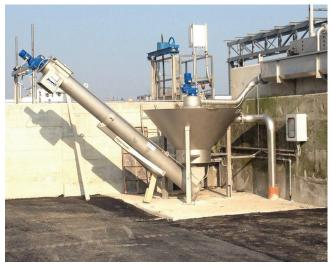
At high level on the hopper, is an outlet flange that allows the lightest material and organics to be discharged.
