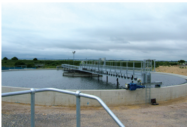
Rotating Full Bridge Scraper
