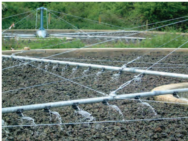
Tubular arms with jet nozzles
