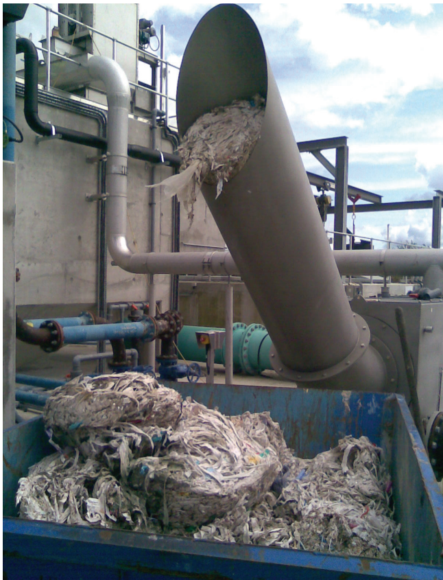
Elevated screenings outlet into a standard skip.
